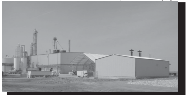
During 2006, Quad County Corn Processors added Golden Bran® storage just east of the process building as well as a new boiler room, on the far right in this photograph.
